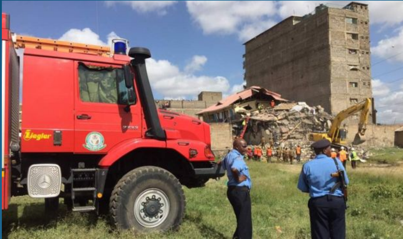
Collapsed Seven –Storey building, Nairobi, Kenya. Source; www.bbc.com/news/world-Africa
