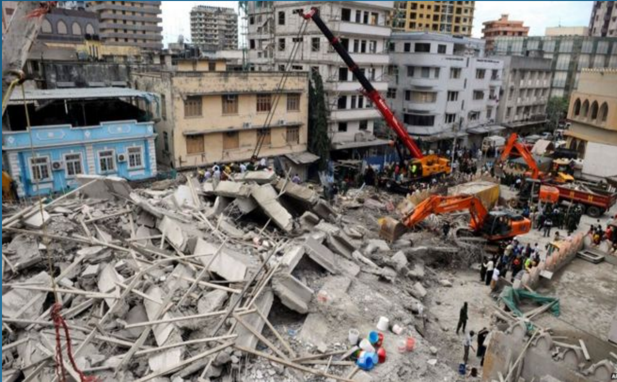
Collapsed Multi -Storey building, Dar es Salaam, Tanzania. Source; www.bbc.com/news/world-Africa
