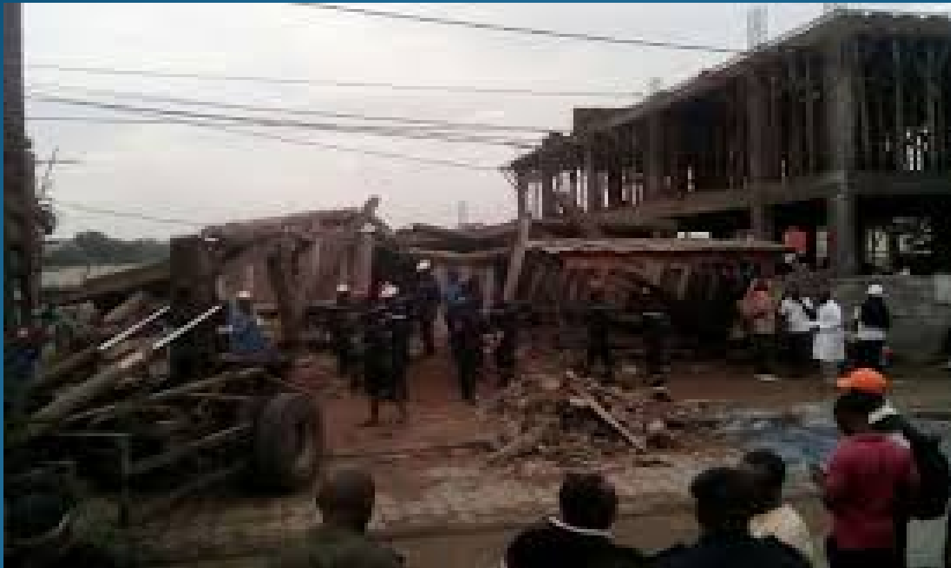
Collapsed two-storey building in Douala, Cameroon. Source; www.today.ng/news/africa/
